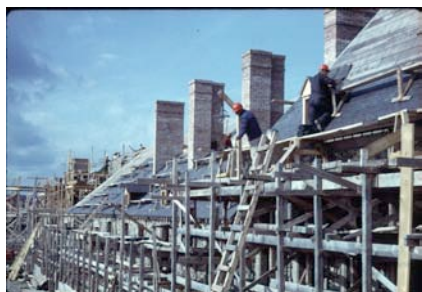
Reconstructing King's Bastion 1960s
